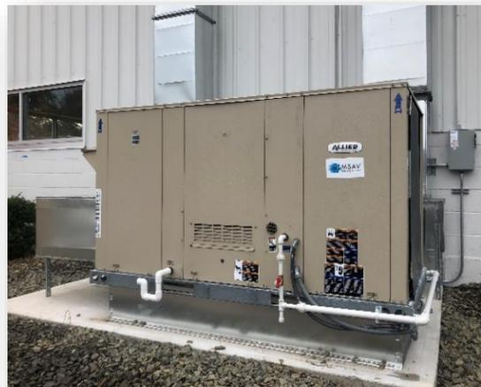
The newly designated KGB and KCB models come with the reheat option and are available from 2 to 25 tons with standard tube and fin coils.
