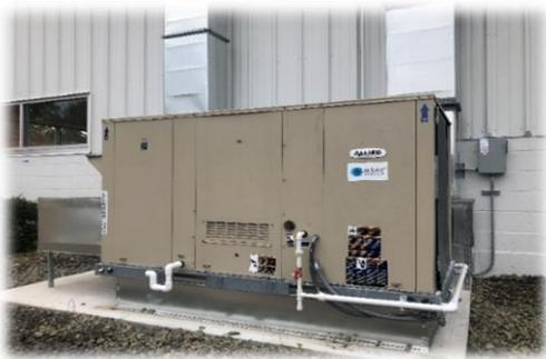
**Allied K-Series™** outdoor, ground-mounted rooftops with horizontal discharge provided heating and cooling to the 10,000 sq.ft. light manufacturing area and 4,500sq. ft. office area.
